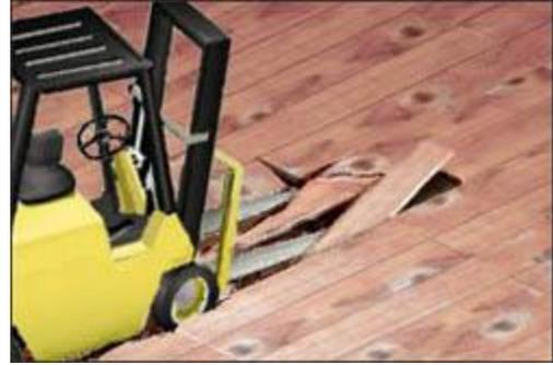
**Figure 5. Forklift weight exceeded the load limit of the flooring.**
